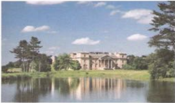
View of the classical Palladian-style house from across the lake
