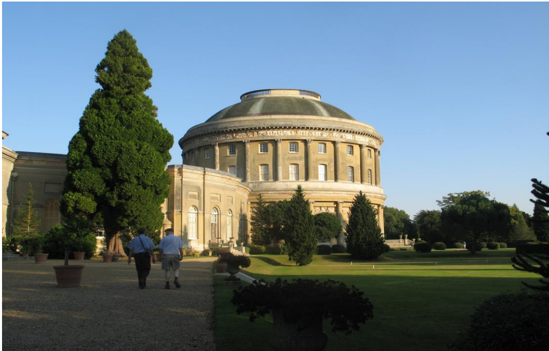
The great Rotunda, Ickworth House. (Photo: Lynne Quayle)
