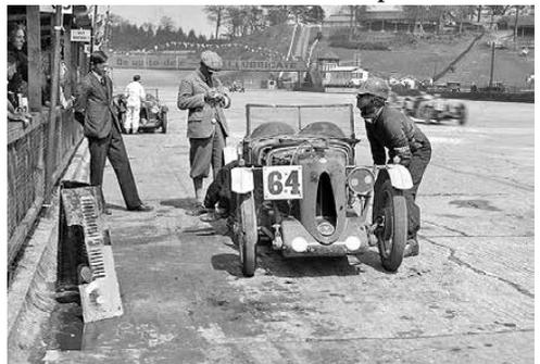
M.G. C type of F.M Montgomery and R Hebler. Retired first day, broken piston.
