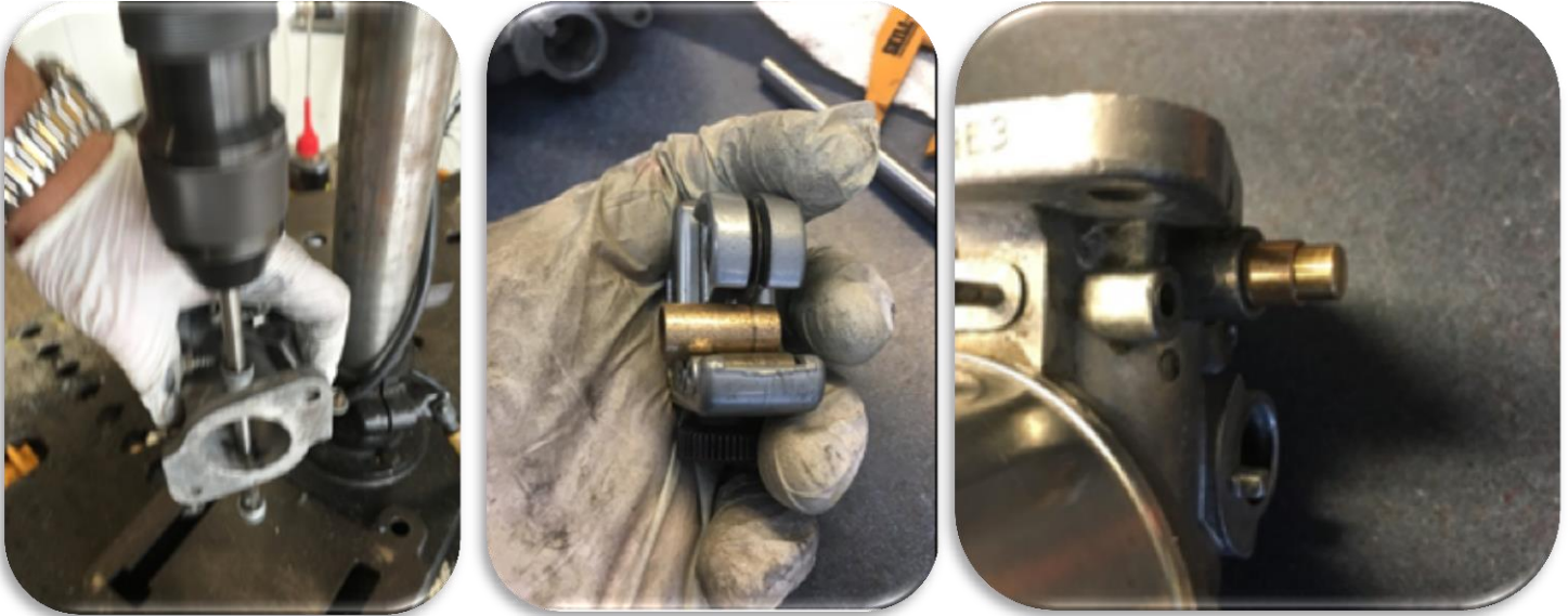
Figure 2. Reaming out an Old Bush; Cutting Down the Inner Bush; and Leaving the Outer Bush Long
